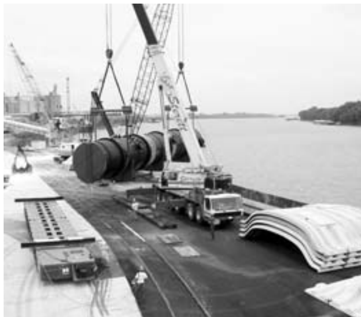
A transload in progress from barge to truck.
